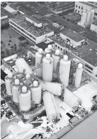
Toppled tanks at a brewery in Sendai, Miyagi Prefecture, northeastern Japan, March 11, 2011
