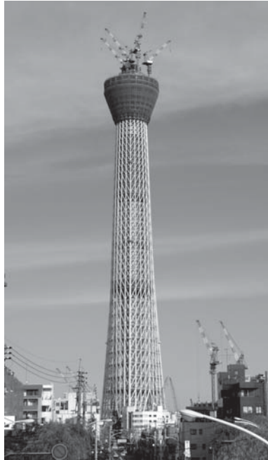
Tokyo Sky Tree under construction
